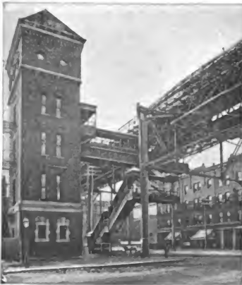
PASSENGER ELEVATOR AND STATION, ELEVATED RAILROAD, EIGHTH AVENUE AND 118TH STREET.
